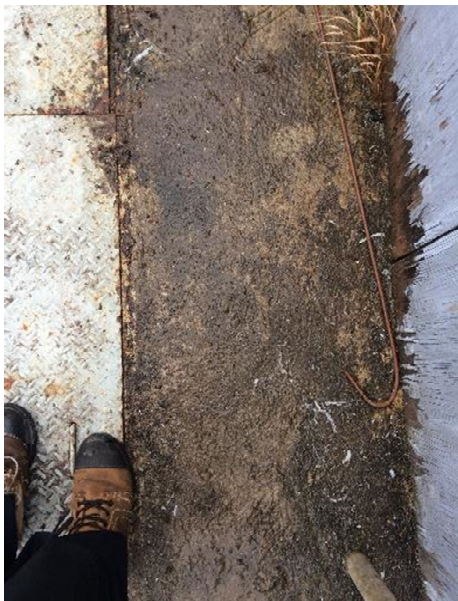
Photo 2 Unit 8 Tailrace Deck - Upstream Side ( 2023-08-22_08h-36mA.jpg )
