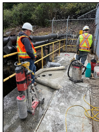
Photo 6 Core 6 location near Corehole 2
