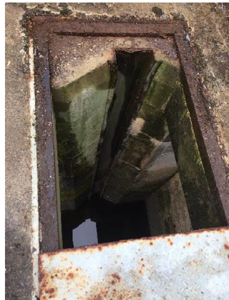
Photo 4 South Gate Slot - Embedded Steel Guide ( 2023-08-22_08h-21m.jpg )
