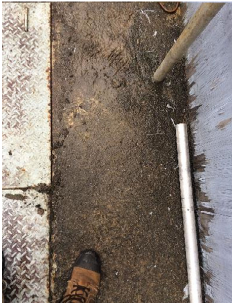
Photo 3 Unit 8 Tailrace Deck - Upstream Side ( 2023-08-22_08h-36mB.jpg )
