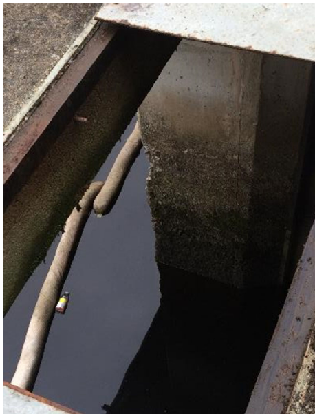
Photo 7 North Gate Slot - View of Center Pier ( 2023-08-22_09h-27mA.jpg )
