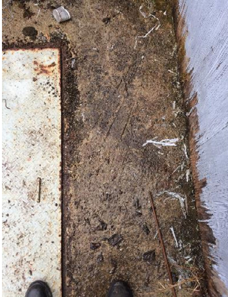
Photo 1 Unit 8 Tailrace Deck - Upstream Side ( 2023-08-22_08h-36m.jpg )
