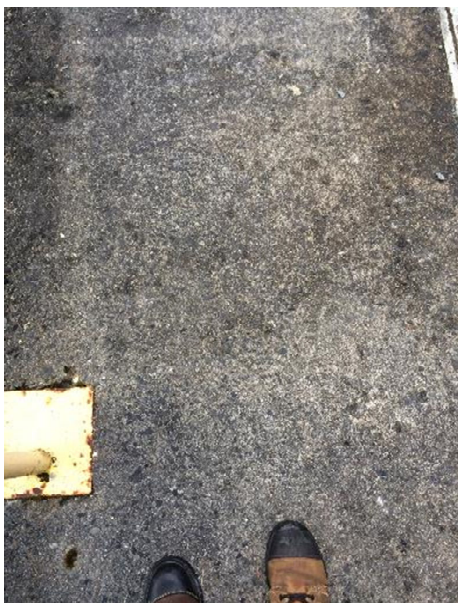
Photo 14 Unit 8 Tailrace Deck - Downstream Side ( 2023-08-22_08h-39mA.jpg )
