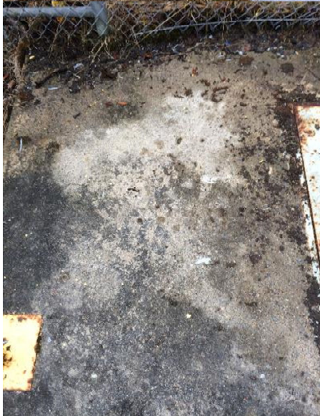
Photo 9 Unit 8 Tailrace Deck - Downstream Side ( 2023-08-22_08h-37mD.jpg )
