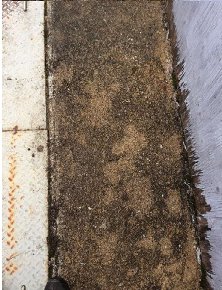
Photo 5 Unit 8 Tailrace Deck - Upstream Side ( 2023-08-22_08h-37m.jpg )
