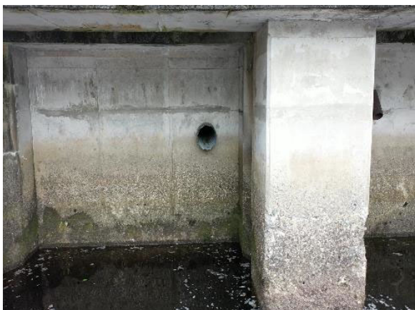
Photo 3 Unit 8 Central Pier between Draft Tube Bays (DJI_0187 - frame at 0m36s.jpg)
