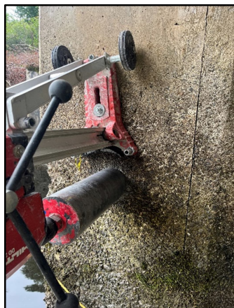
Photo 5 Coring drill setup at Core 5 location, NE side of central column
