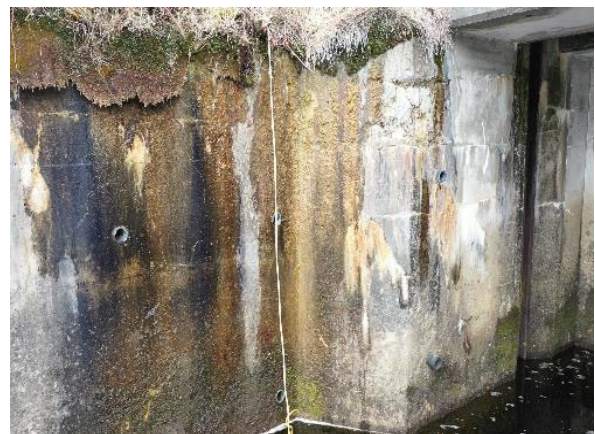
Photo 4 Unit 8 South Wingwall (DJI_0187 - frame at 0m38s.jpg)
