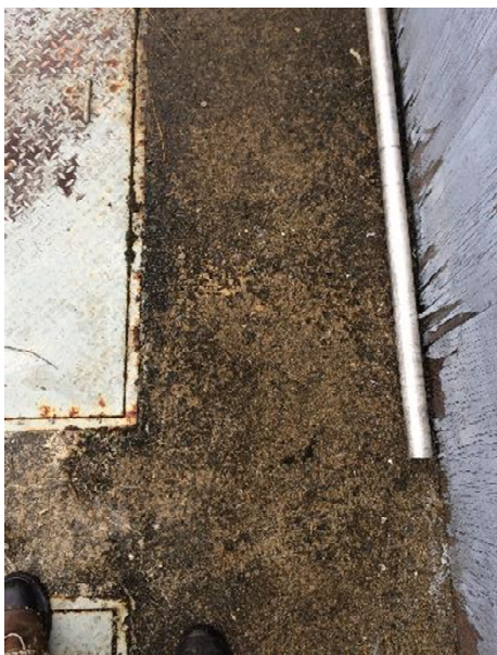
Photo 4 Unit 8 Tailrace Deck - Upstream Side ( 2023-08-22_08h-36mC.jpg )
