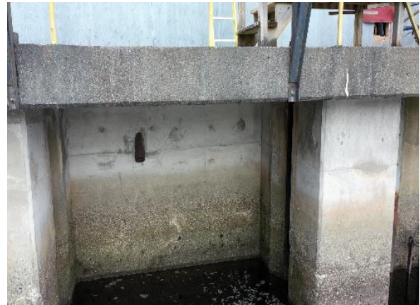
Photo 2 Unit 8 South Draft Tube Bay (DJI_0187 - frame at 0m19s.jpg)
