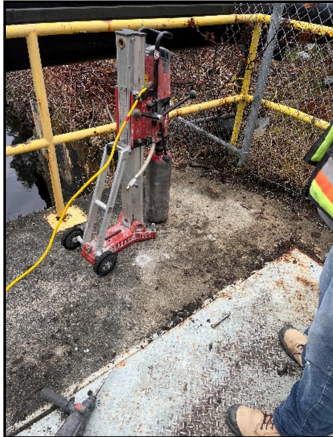
Photo 1 Core 1 location, SW side of Draft Tube Deck
