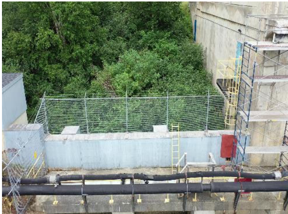
Photo 1 Unit 8 Tailrace Deck (from above) (DJI_0187 - frame at 0m0s.jpg)
