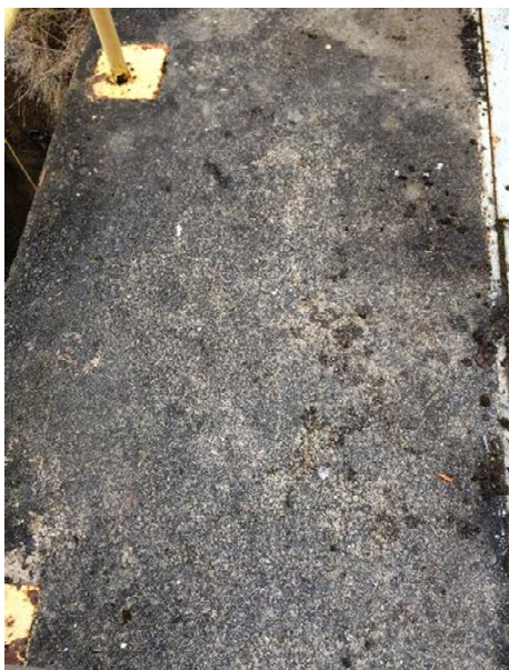
Photo 10 Unit 8 Tailrace Deck - Downstream Side ( 2023-08-22_08h-38m.jpg )
