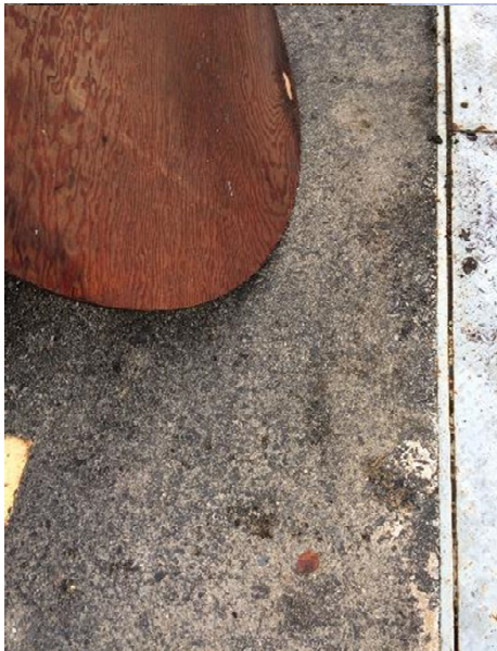
Photo 11 Unit 8 Tailrace Deck - Downstream Side ( 2023-08-22_08h-38mA.jpg )
