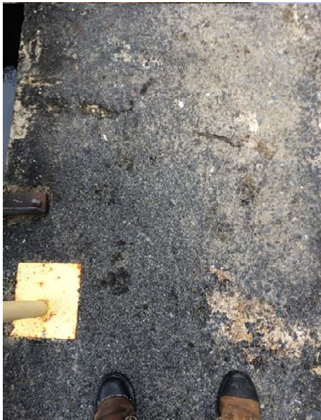
Photo 13 Unit 8 Tailrace Deck - Downstream Side ( 2023-08-22_08h-39m.jpg )
