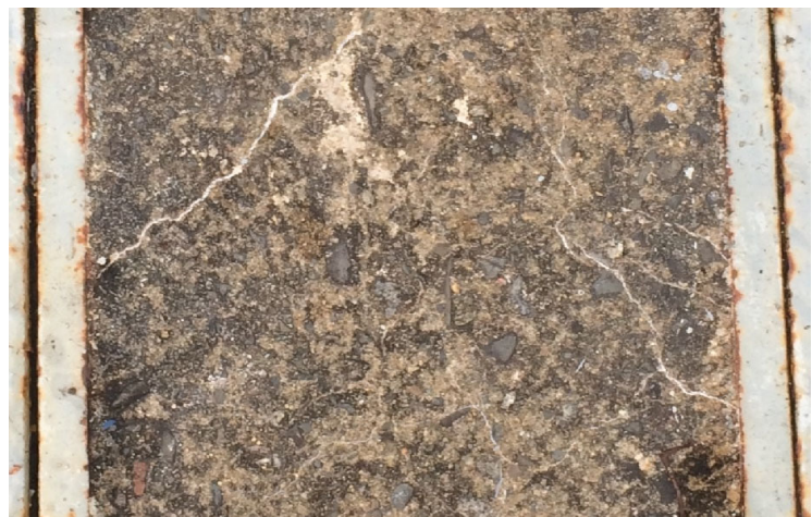
Closeup of concrete between gate slots
