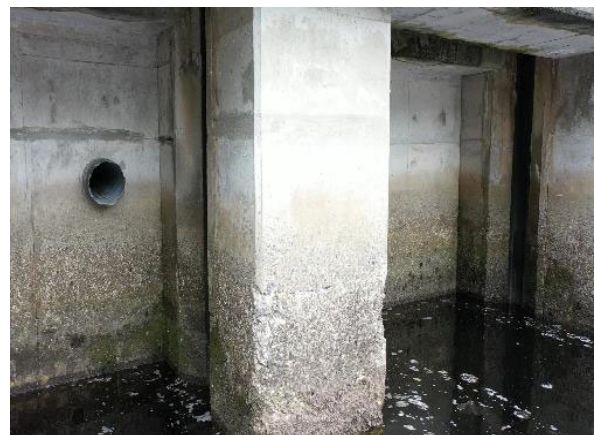
Photo 6 Unit 8 Central Pier (DJI_0187 - frame at 1m36s.jpg)
