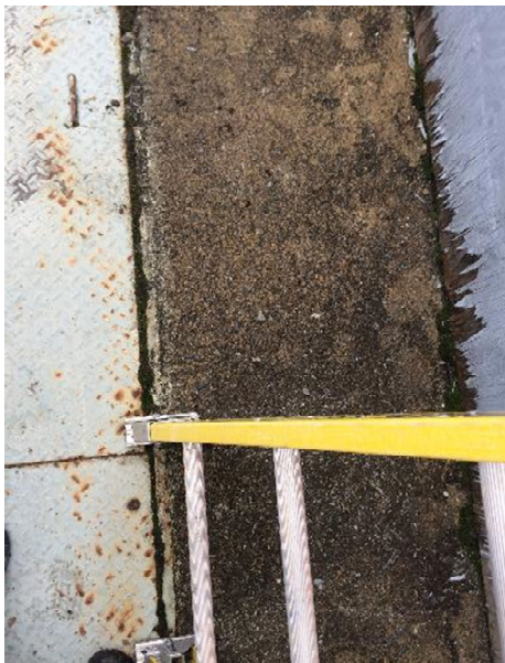
Photo 6 Unit 8 Tailrace Deck - Upstream Side ( 2023-08-22_08h-37mA.jpg )
