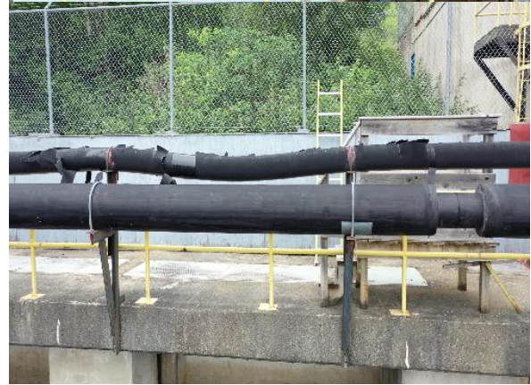
Photo 8 Unit 8 Side View of Deck Slab (DJI_0187 - frame at 2m15s.jpg)
