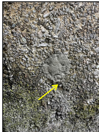
Photo 4 Repaired corehole at Core 4 location, SW side of central column
