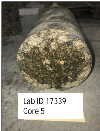
Photo 15 Core 5 exposed surface
