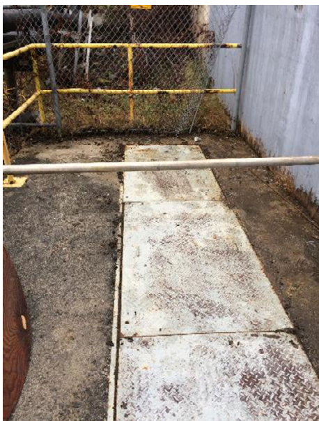
Photo 12 Unit 8 Tailrace Deck - Downstream Side ( 2023-08-22_08h-38mB.jpg )
