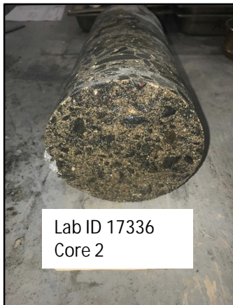
Photo 9 Core 2 exposed surface
