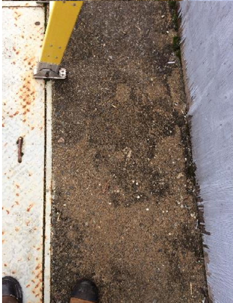
Photo 7 Unit 8 Tailrace Deck - Upstream Side ( 2023-08-22_08h-37mB.jpg )
