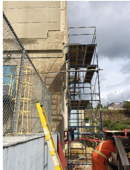
Photo 2 View looking South towards Unit 7 ( 2023-08-21_12h-26m.jpg )
