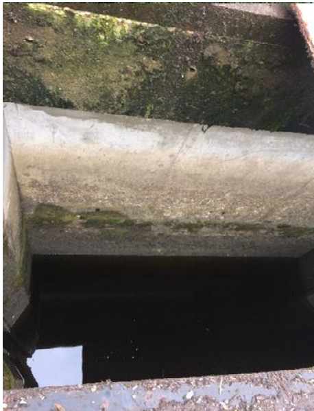
Photo 5 South Gate Slot - View of Back Wall ( 2023-08-22_08h-21mB.jpg )
