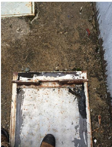
Photo 8 Unit 8 Tailrace Deck - Upstream Side ( 2023-08-22_08h-37mC.jpg )
