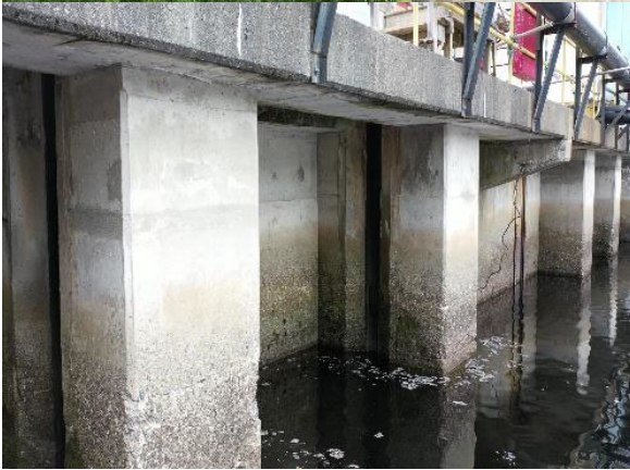
Photo 7 Unit 8 Looking Towards Unit 7 (DJI_0187 - frame at 1m9s.jpg)
